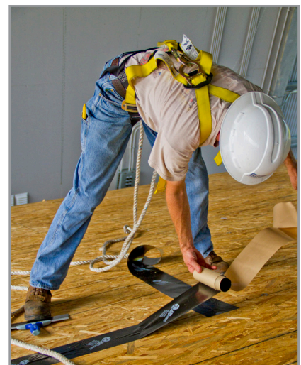
Sealing the roof deck
